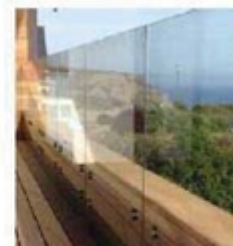
3. Recessed glazed balustrade, not visible from street level of surrounding 5th & 6th floor balconies
