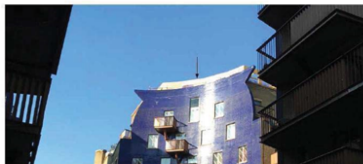
Site progress under NMA 15/AP/0060
