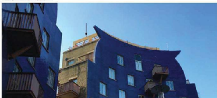
Site progress under NMA 15/AP/0060
